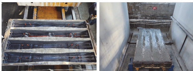
Figure 6 Smart and ordinary sleepers before and after concrete pouring
