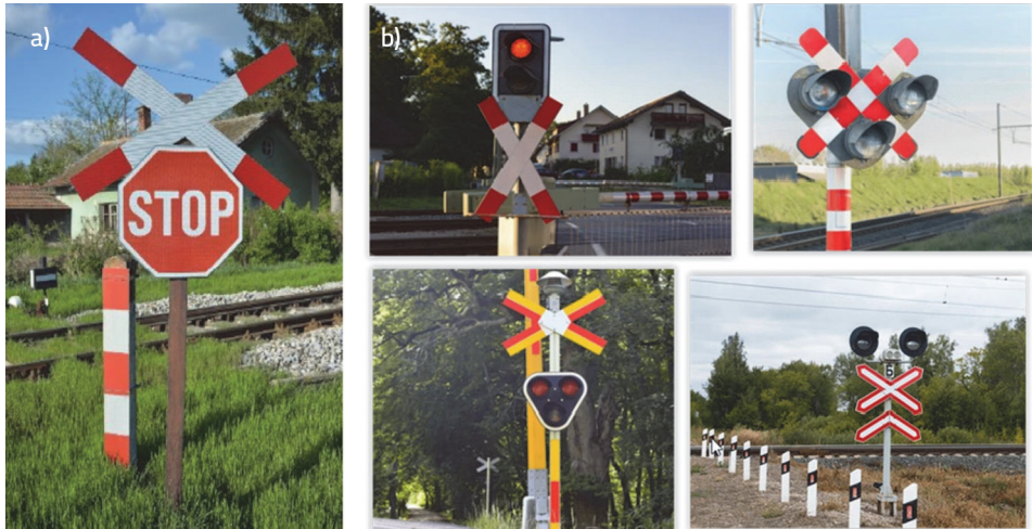
Figure 1 a) Marking of crossing with A37 and B02 signs in Croatia; b) some EU countries
