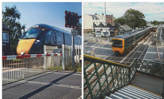
Figure 4 Crossing secured with bumpers plus light-sound, pedestrian crossing levelled by a guardrail (British Railways) [13]
