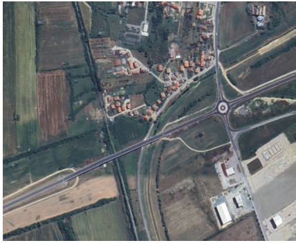
Figure 3 View of the constructed Pruga bridge and Cerik roundabout [1]
