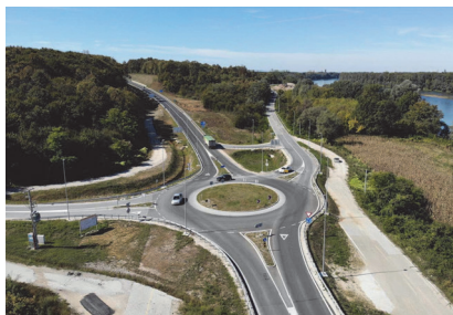
Figure 2 View of the constructed Gređice roundabout [2]
