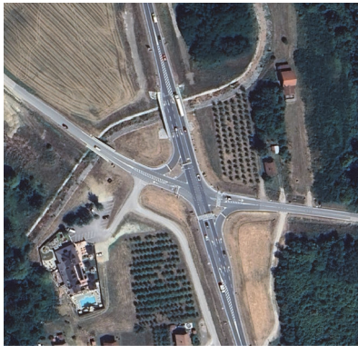
Figure 4 View of the constructed Ulice at-grade junction [1]
