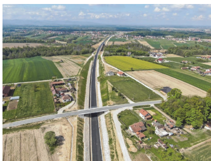
Figure 6 View of the constructed overcrossing Ražljevo [2]
