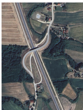
Figure 7 View of the constructed overcrossing Grbavica [1]
