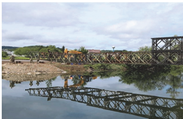
Figure 4 Bailey bridge abutment
