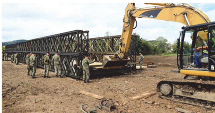
Figure 5 Bailey bridge launching
