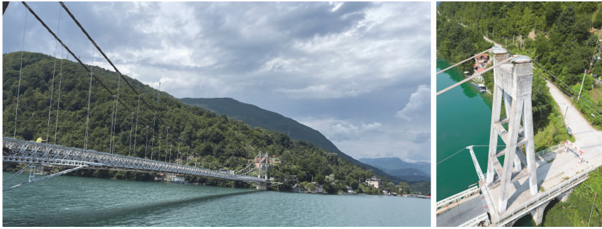
Figure 1 View of the suspension bridge in Ostrožac
