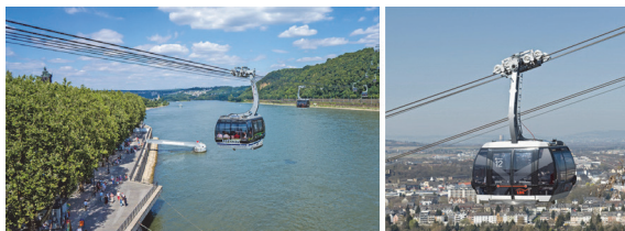
Figure 5 Seilbahn Koblenz gondola [19]
