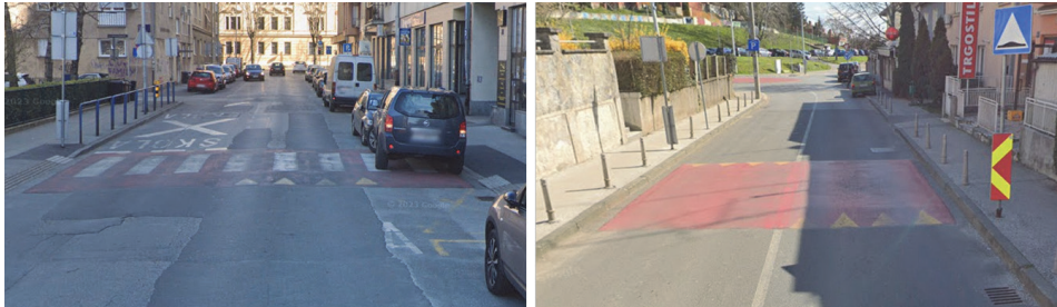
Figure 3 Red-coloured speed hump installed across the entire width of the carriageway at: a) location L1, b) location L2
