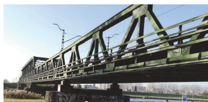
Figure 2 The steel riveted superstructure of the railway bridge over the Oder River in Opole
