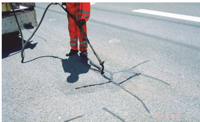
Figure 1 Crack sealing with bituminous sealing compound
