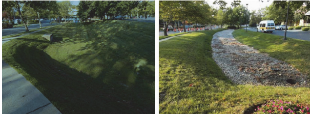
Figure 2 Dry retention basin with a spillway and drainage ditch in the urban area [9]
