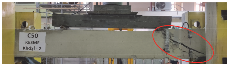
Figure 3 Development of shear cracks in the beam
