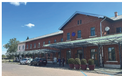
Figure 6 Osijek railway station after the reconstruction, 2024.
