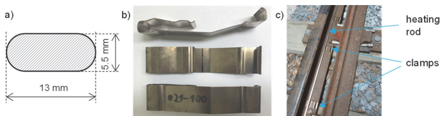
Figure 1 a) Common cross section of heating rod; b) Uninstalled heating rod clamp; c) Installed heating rod with clamps at the foot of the stock rail
