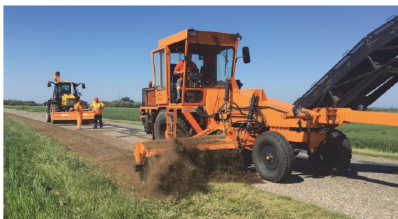
Figure 3 Madro SP-1500 shoulder milling machine in work (Photo: Csaba Tóth)
