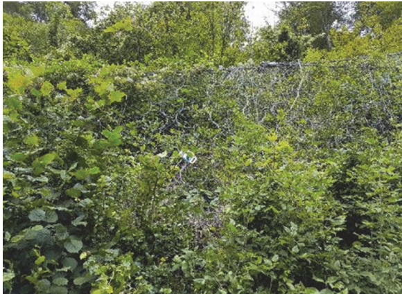
Figure 6 Rockfall protection barrier disappearing into the vegetation
