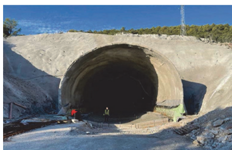
Figure 3 Breaking of the Supava tunnel [4]
