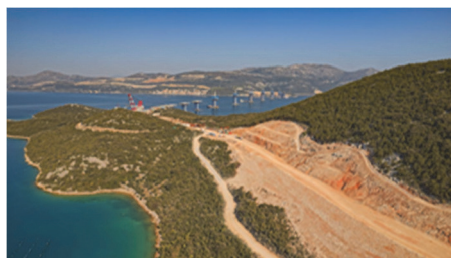
Figure 2 Access road penetration process [4]
