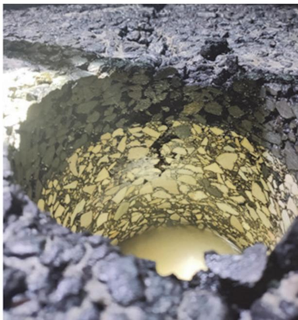
**Figure 3** Top-down crack observed during the coring campaign
