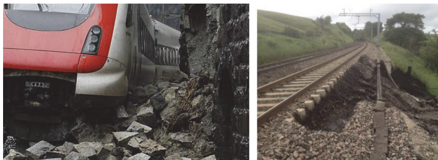
Figure 5 Dangerous situations on railway tracks: collapsed stones (left) and teared off super/substructure (right)
