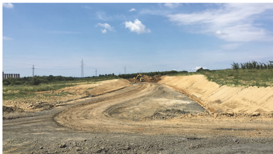
Figure 2 Railway soil-subgrade preparation, 12/06/2021
