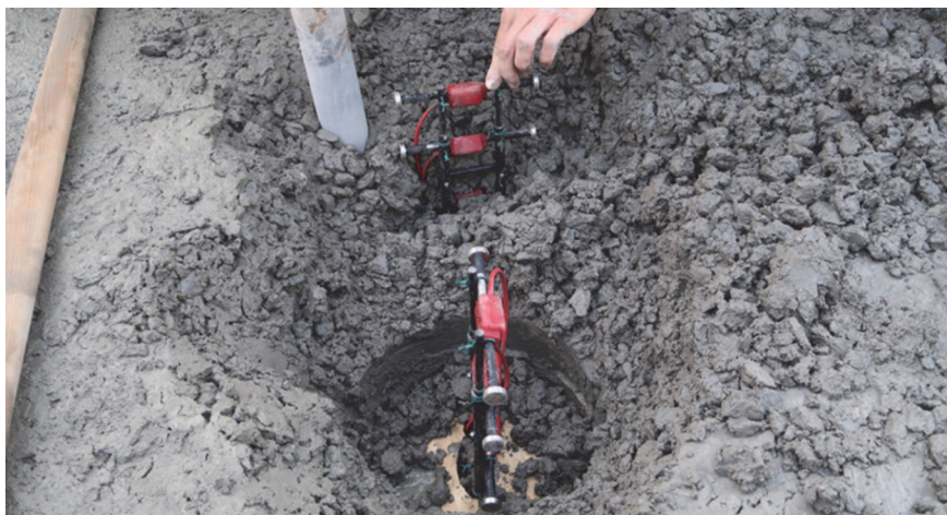
Figure 1 Placement of gauges (Photo: S. Šulc)
