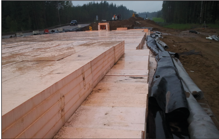
Figure 7 The construction of the lightweight embankment which consists of expanded polystyrene
