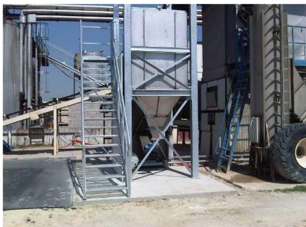
**Figure 2** Automated feeding of the additive (Plant CIFA Mityr-Mory, France)
