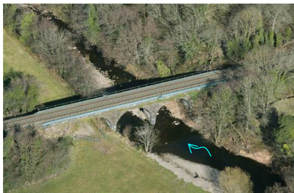
Figure 4 Aerial view of UB18 bridge, looking upstream.
