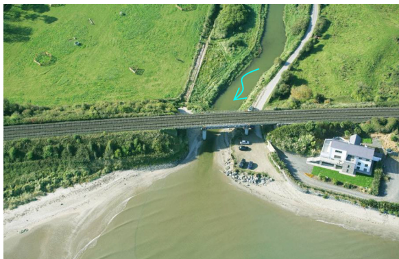
Figure 2 Aerial view of UB65 bridge, looking upstream
