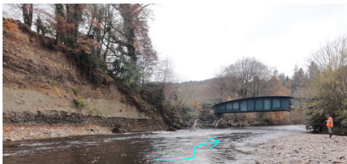
Figure 3 Upstream river channel at UB207 bridge, looking downstream
