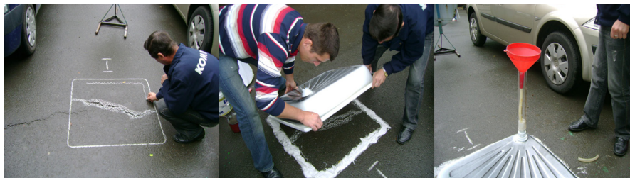
Figure 4 Surface marking; Sealing material application; Field device
